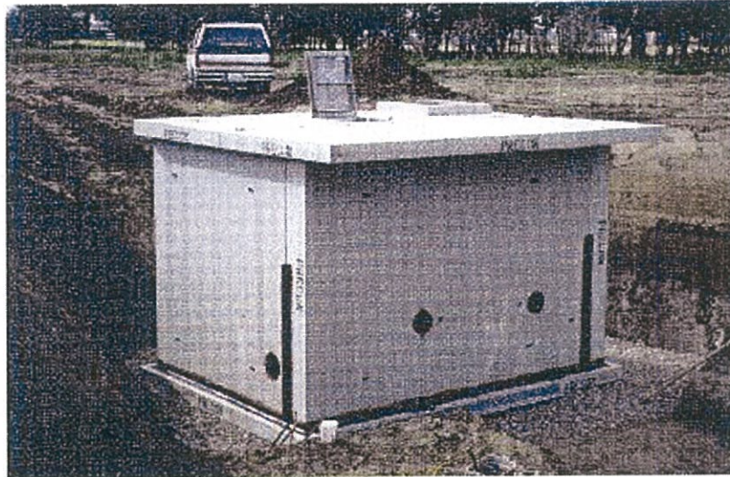
STANDARD WELL WELL LIFT STATION
